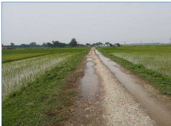
Figure No 5.1: Urban Road Condition at Ward 5
